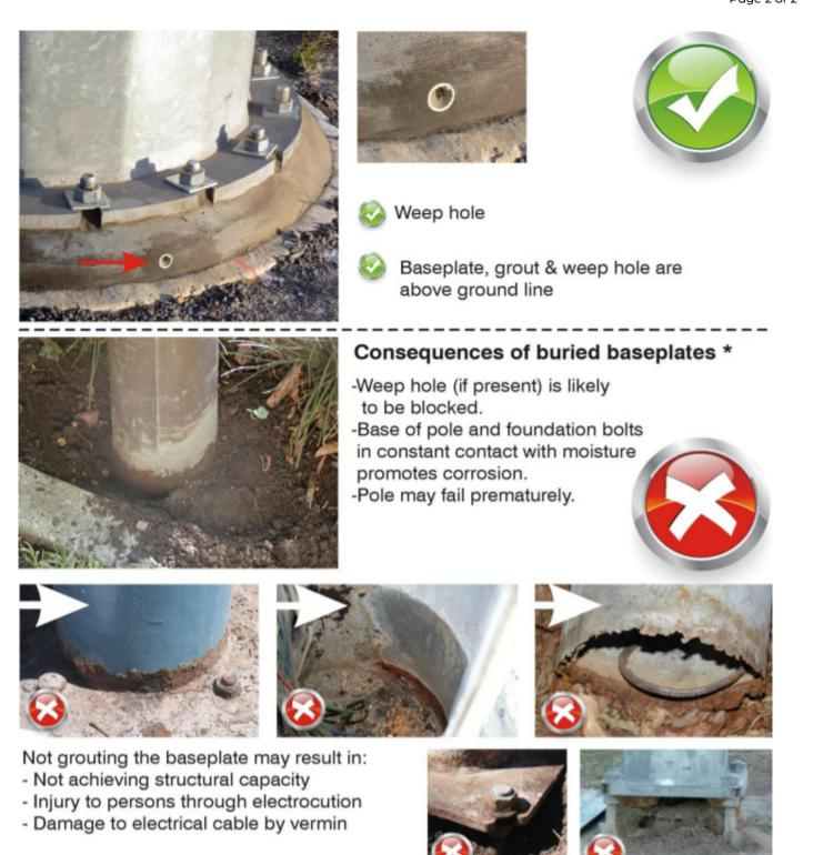
\*Note: in rare circumstances pole bases are intentionally buried (eg. pedestrian malls etc.) The designer will need to ensure that the method of burial is sufficiently detailed to ensure the pole and foundation bolts are protected to prevent corrosion.
